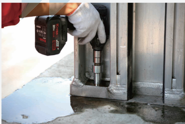
3 鎖緊緊固螺栓
